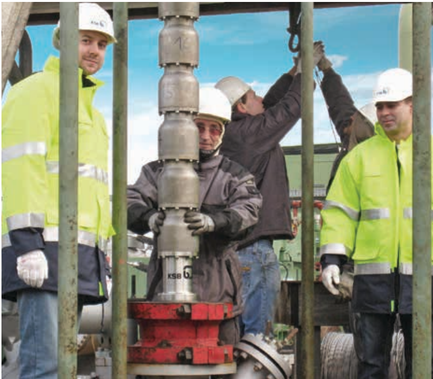
Installation on site
