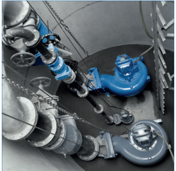
Fig. 53: Vertical valve arrangement in the pump sump
