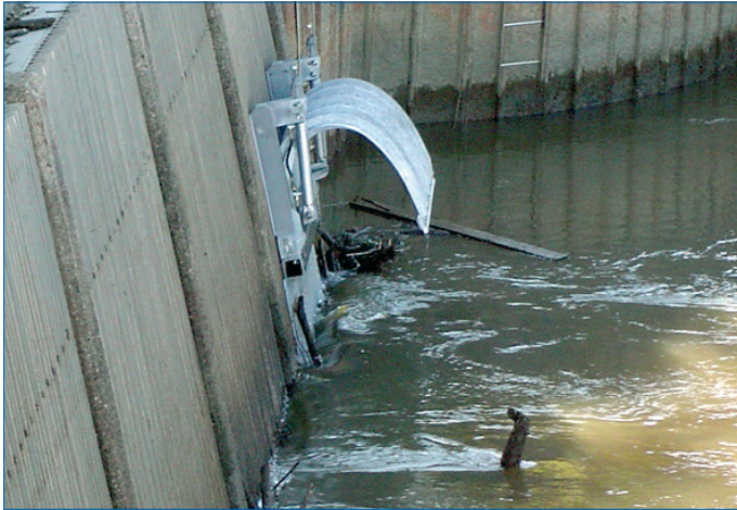
Fig. 85: Screen with automatic cleaning system
