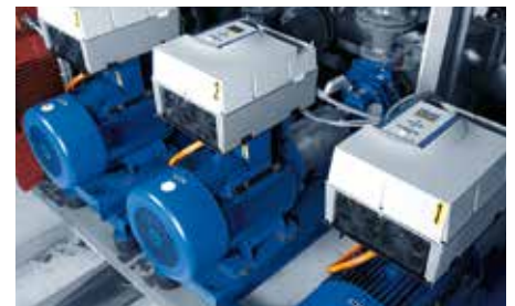
Each pump is designed for a flow rate of 100 m³/h.
