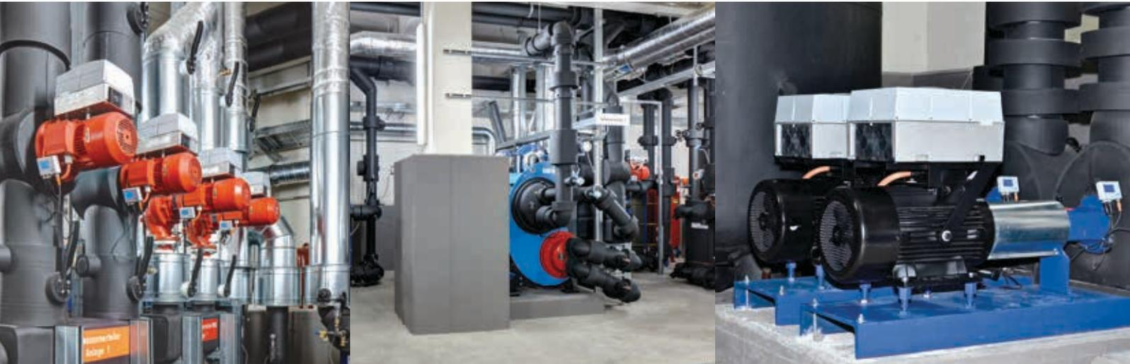
The KSB pumps from the Etanorm or Etaline range are employed in pairs of two. They are operated in parallel under part-load conditions, with each individual pump being capable of producing around 80 % of the required maximum output. This is cheaper in terms of energy than using a single larger pump. Although a single pump could produce the total
