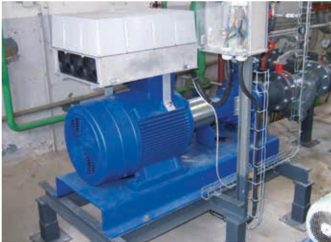
Etanorm 80-200 with motor-mounted PumpDrive
