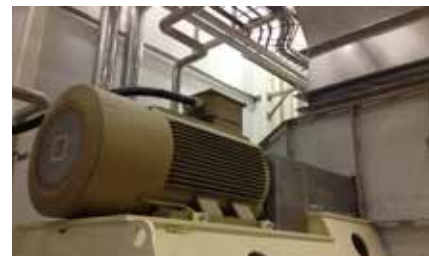
Energy efficiency / power quality systems
