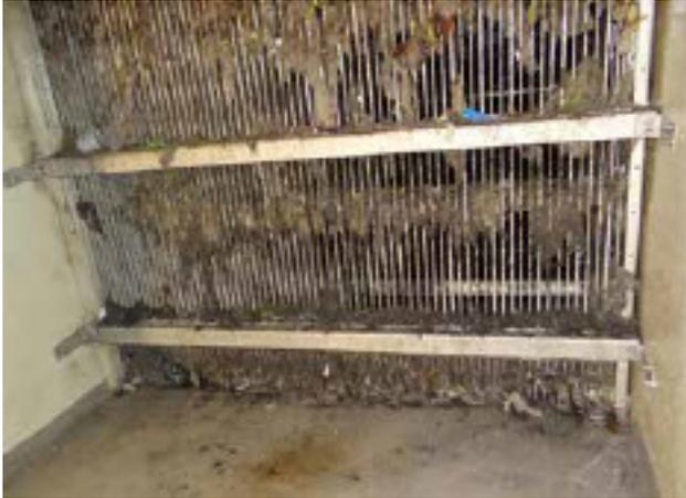
Image 1. A bar screen is loaded with “flushable” products. (Images and graphics courtesy of KSB Inc.)
