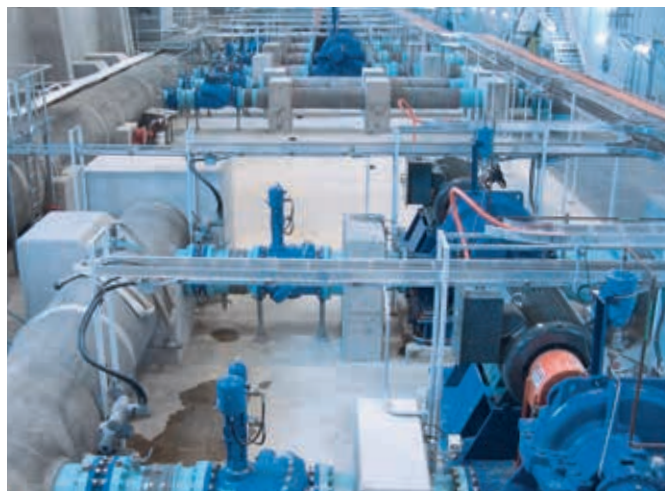
Beckett Sproule Pumping Station
